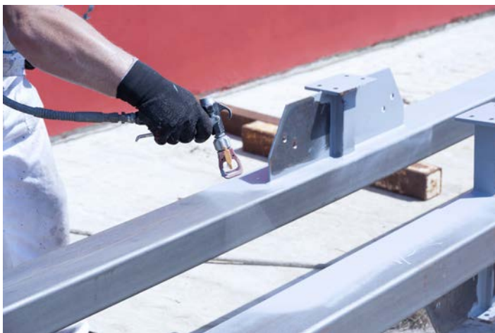
VpCI® coating application
